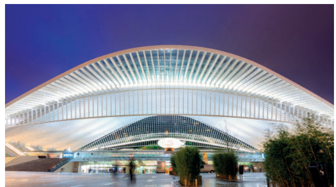
Liège-Guillemins railway station - Liege (Belgium)
