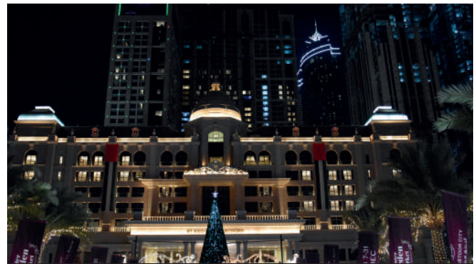
The St. Regis - Dubai (United Arab Emirates)
