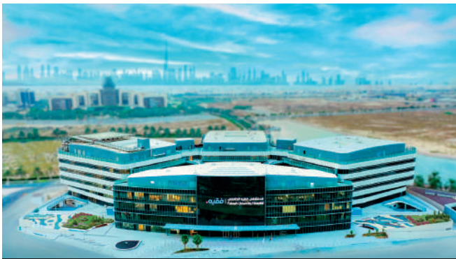
Fakhri Hospital - Dubai (United Arab Emirates)
