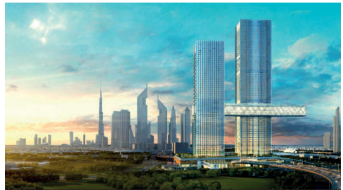
One Za'abel Project - Dubai (United Arab Emirates)
