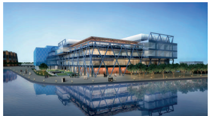
Arzanah Hospital - Abu Dhabi (United Arab Emirates)
